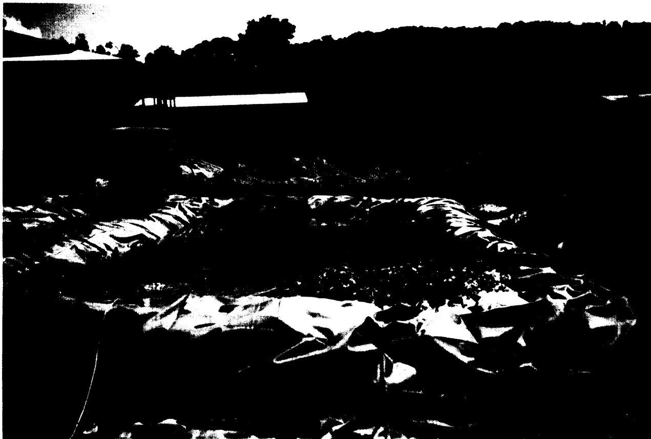
This plastic lined settling pond is part of the small-scale biogas system in the Northern Mariana Islands. The effluent from the pond is discharged through an irrigation system.
