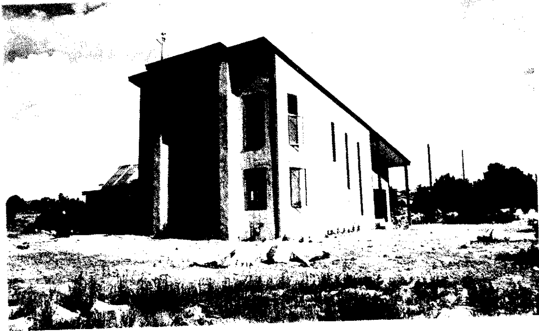
Figure 53.—This Home in Los Alamos, N. Mex., Combines a Large Trombe Wall With Small Direct Gain Windows and a Rock Storage Bed. The Interior of the Trombe Wall is a Distinctly Attractive Part of the Living Room
