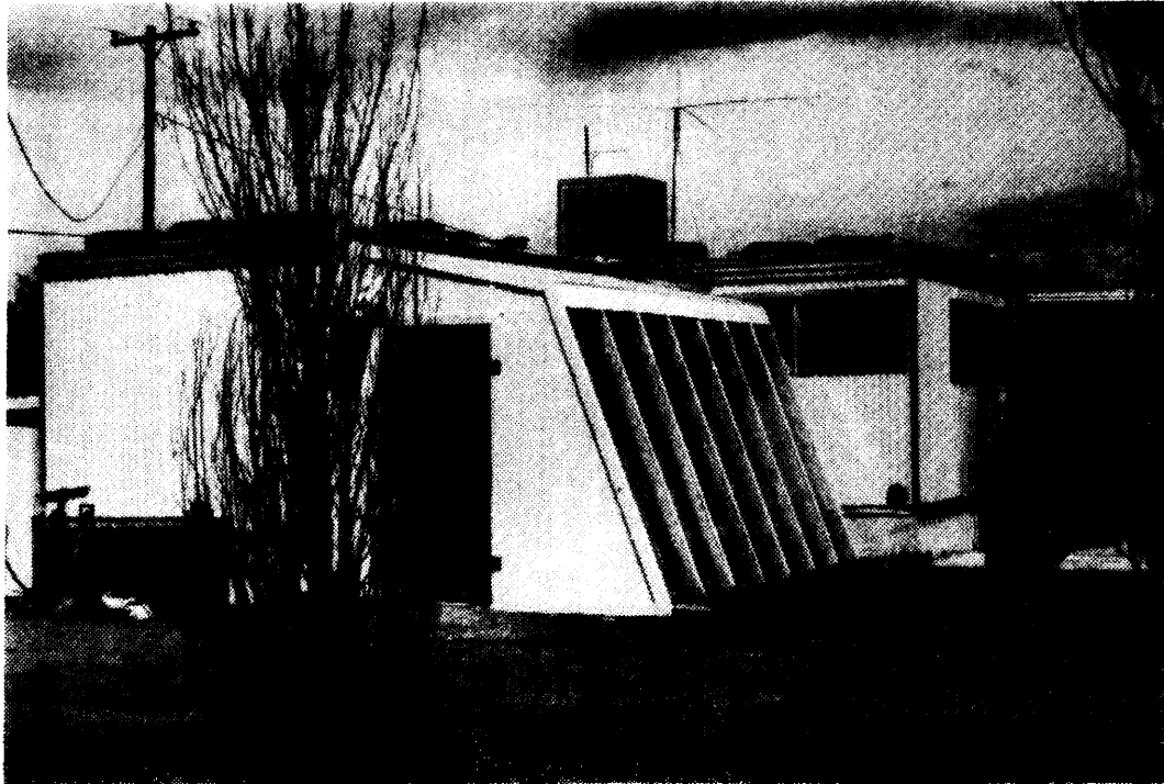
Figure 51 .—This Retrofit Greenhouse is an Example of Those Built by the Solar Sustenance Project
