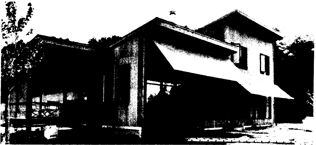
Figure 47.—The Crosley House in Royal Oak, Md., Combines a Trombe Wall System With Direct Gain and a Massive Floor, to Provide 50 to 60 Percent of Its Heating-Needs
