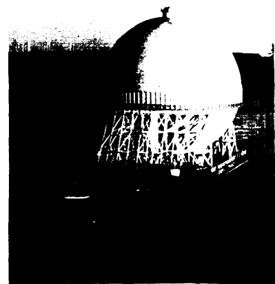
Liquefied natural gas tankers constructed by General Dynamics use five spherical tanks of about 25,000 cubic meters each. Tanks for the ships are constructed in South Carolina and towed by barge to the shipyard at Quincy, Mass., where they are mounted into the ship hull.
