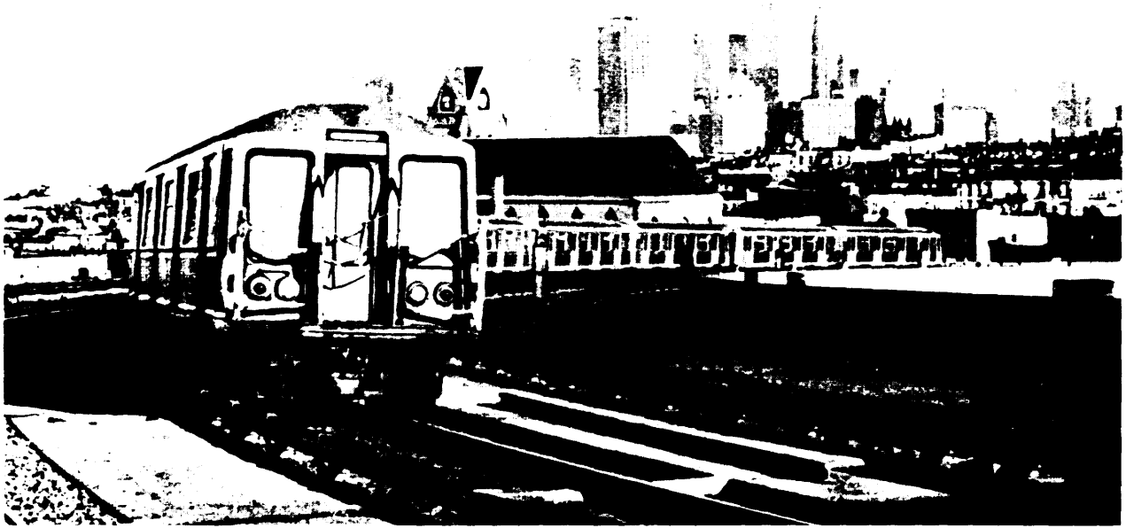
FIGURE 37.—IND F Train on Elevated Line in Brooklyn
