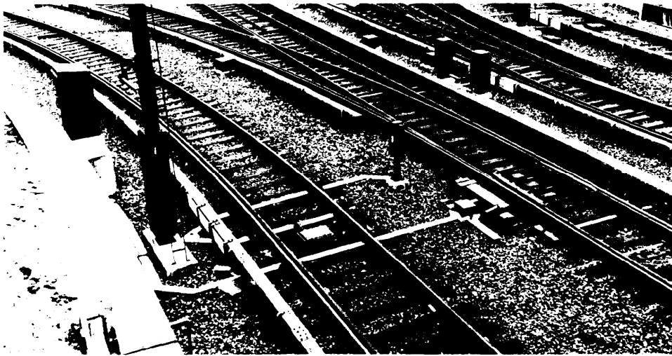
FIGURE 16.—Track Apparatus at an Interlocking
