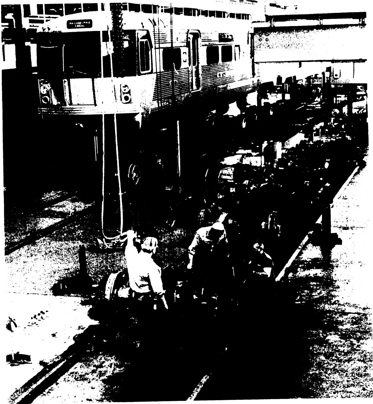
FIGURE 23.—Rail Rapid Transit Car Maintenance Shop
