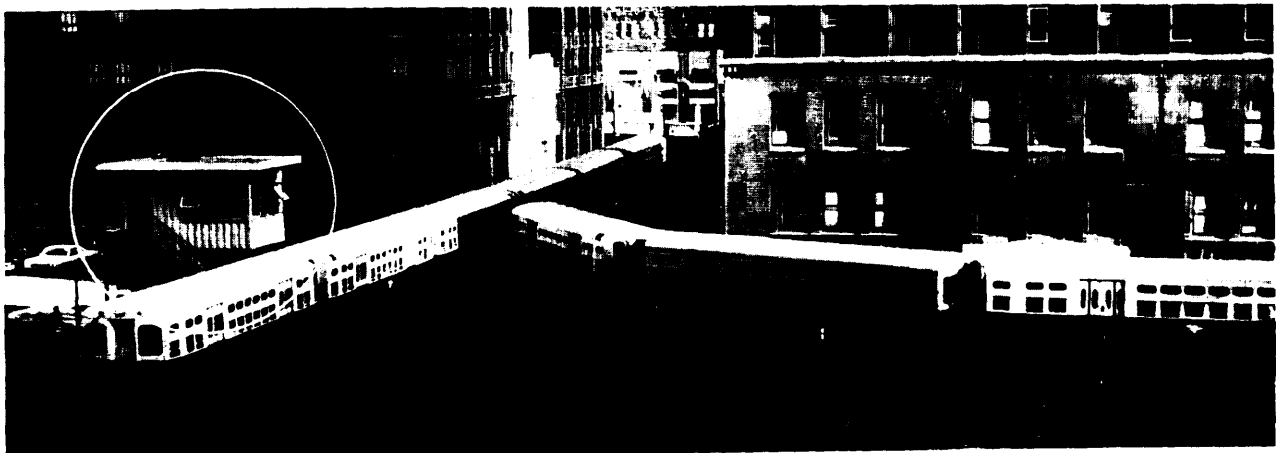
FIGURE 47.—Interlocking Control Tower for Train Protection
