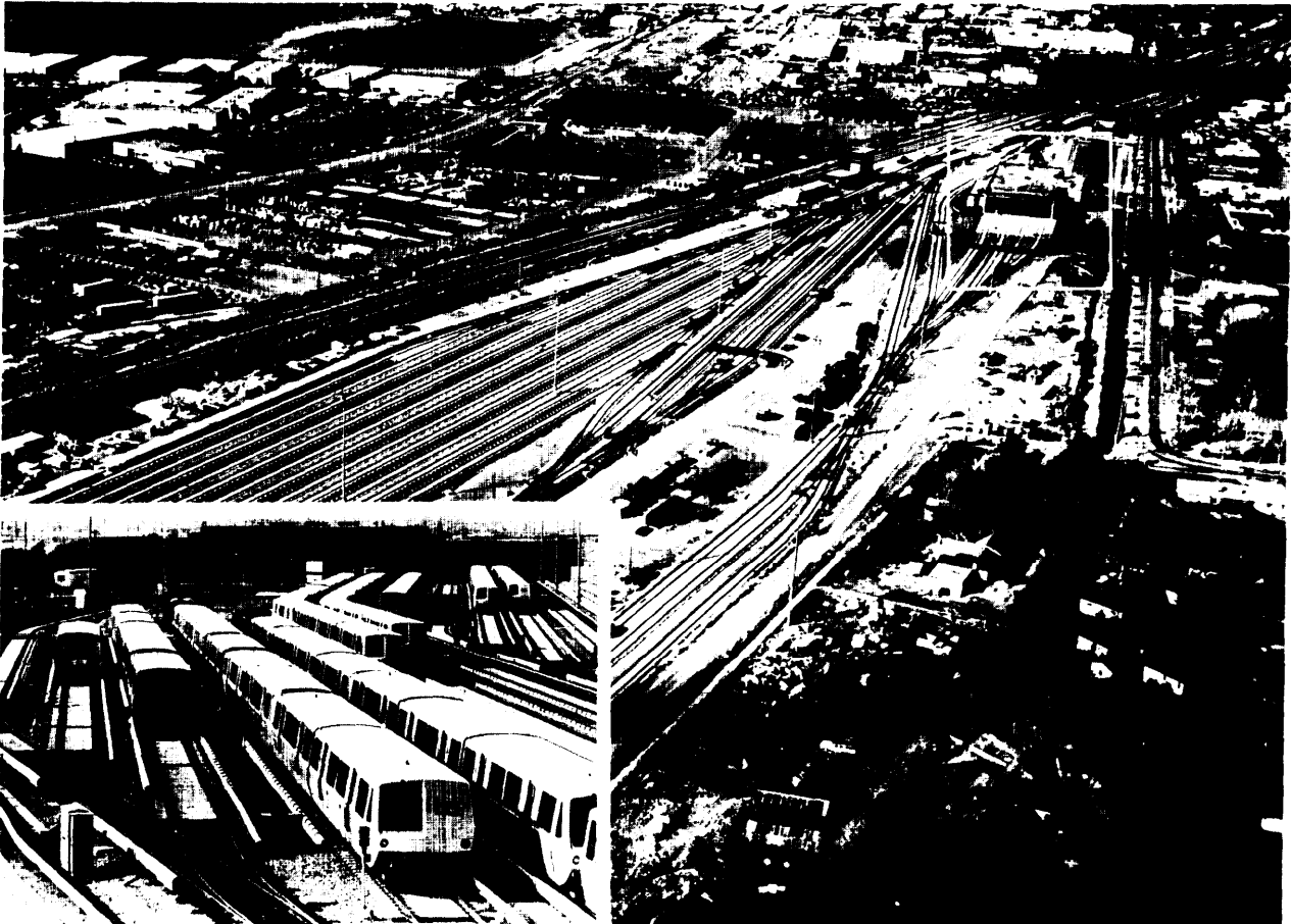
FIGURE 22.—Aerial View of Rail Rapid Transit Yard and Maintenance Facility
