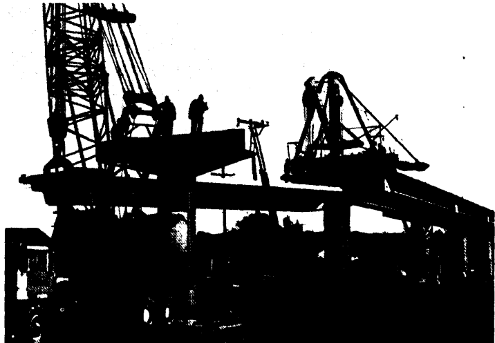
BART Elevated Guideway
