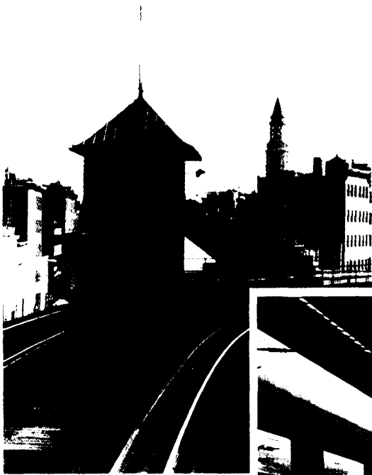
Tower C, at one time the busiest control and interlocking tower in the MBTA system, now replaced by a modern automated facility.
