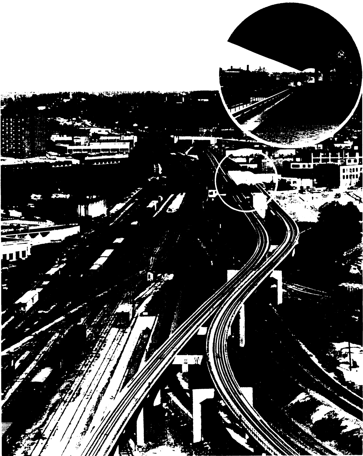
Poor coordination between transit systems and adjacent development leads to situations such as this one at the Washington, DC., Metro's Rhode Island Avenue station. Residents of the housing complex on the left have no direct access to the station.
