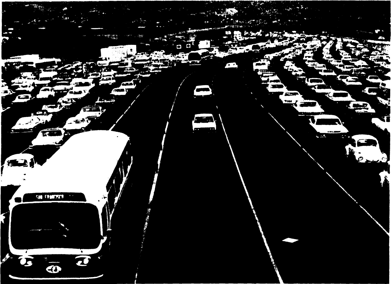
Exclusive Bus and Carpool Lanes on San Francisco-Oakland Bridge
