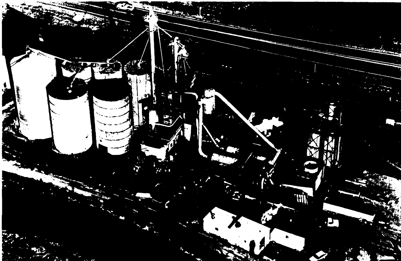
Figure 13.—Aerial View of the Valley Dehydrating Co., Sterling, Colo.
