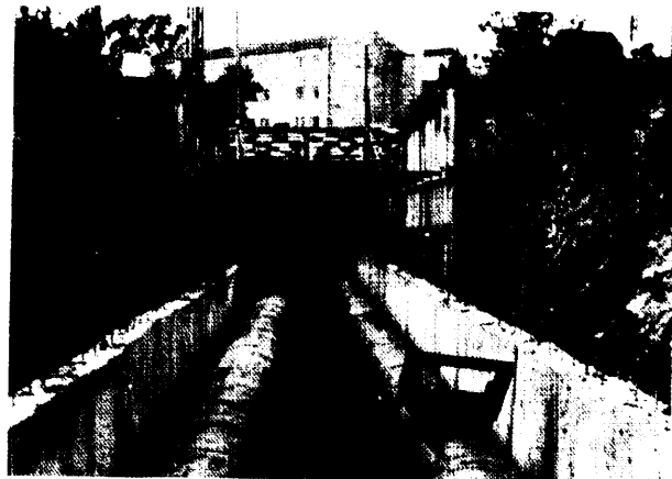
e) High-temperature district heating pipe during construction
