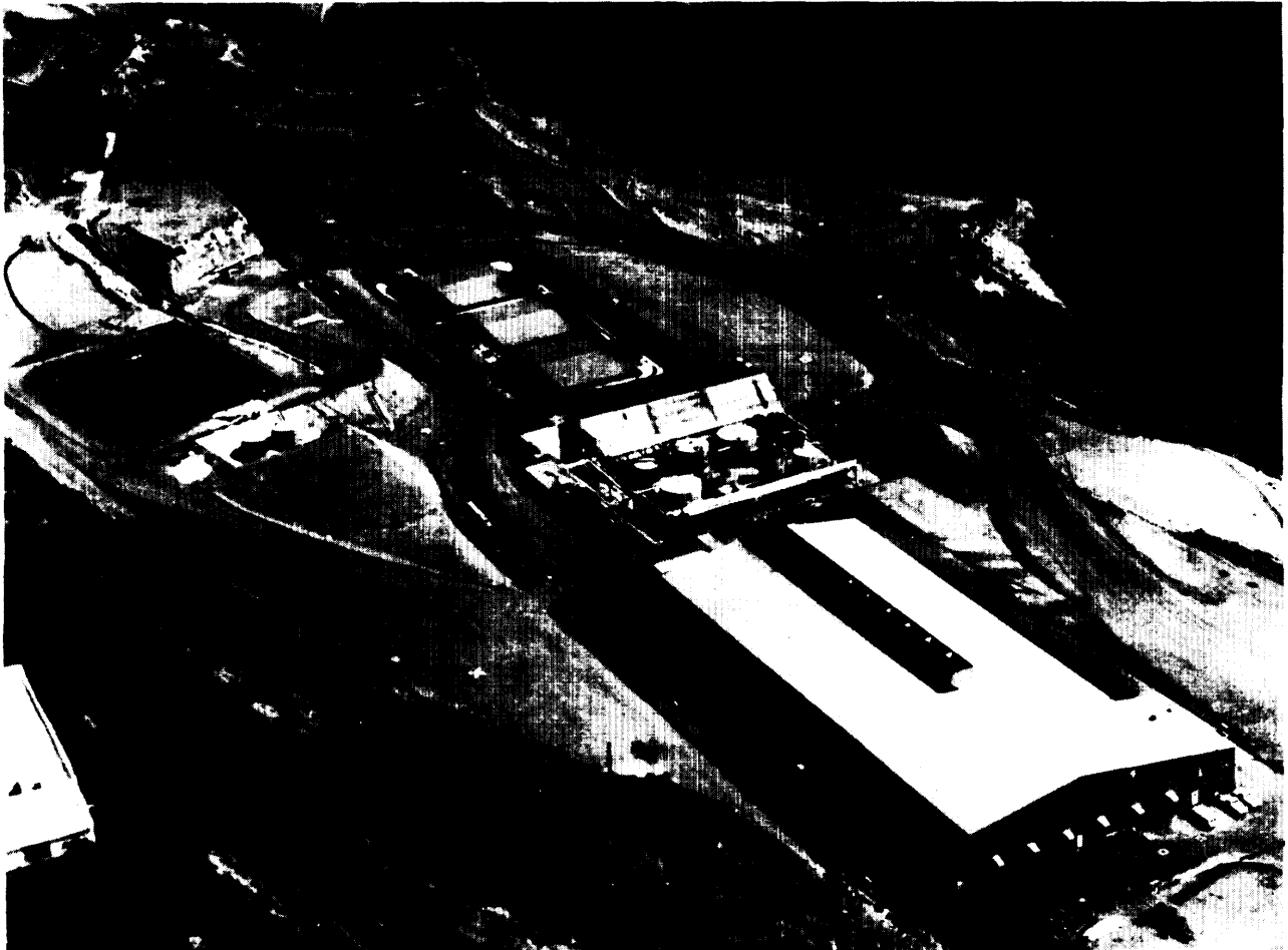
Photo credit Manley-Prim Photography, Tucson, AZ
