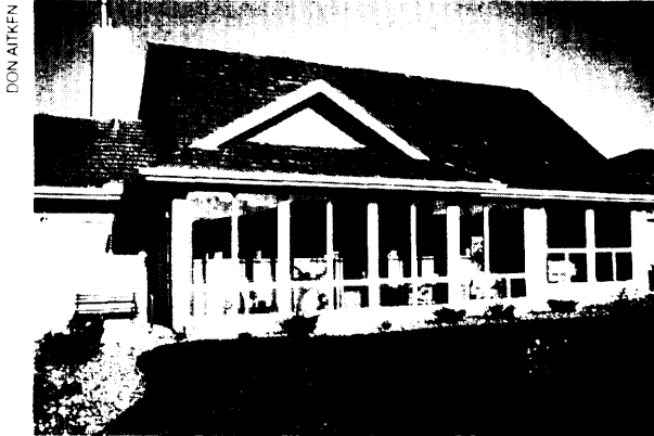
Neuffer Construction homes in Reno, Nevada, use passive design techniques to reduce energy use by 35 to 50 percent compared with conventional homes
