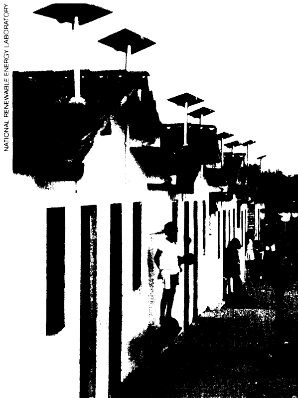
In the state of Ceara in northeast Brazil, all the homes in the village of Cacimba have been outfitted with 50-W PV solar home power systems that provide up 4 to 6 hours of light each night from two fluorescent lights
