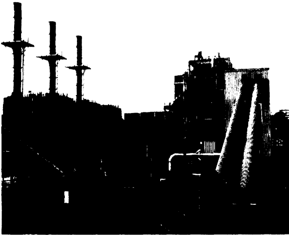
Wheelabrator biomass electric plant in Mt. Shasta, California.
