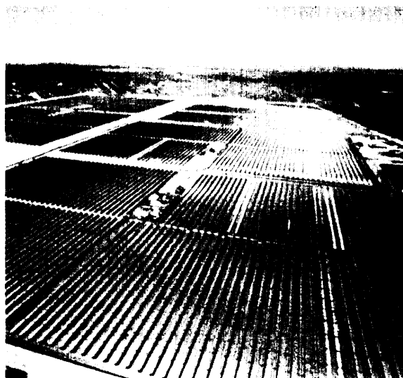
Solar thermal-natural gas hybrid electricity-generating system in the Mojave desert, California.
