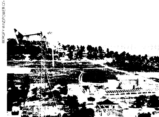
Six 10-kW wind turbines from Bergey Windpower, an 11.2-kW photovoltaic array from Siemens Solar, and a diesel power backup provide power for 150 homes in the village of Xcalac in Quintana Roo province, Mexico.
