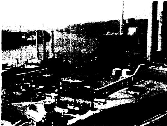
*Ohio Power Co. Tidd Plant, Brilliant, Ohio. Pressurized fluidized bed combustion is one of a variety of technologies being demonstrated under DOE'S Clean Coal Technology Program. Clean coal technologies may have growing markets as coal-dependent countries **around** the world address environmental **concerns**.*
