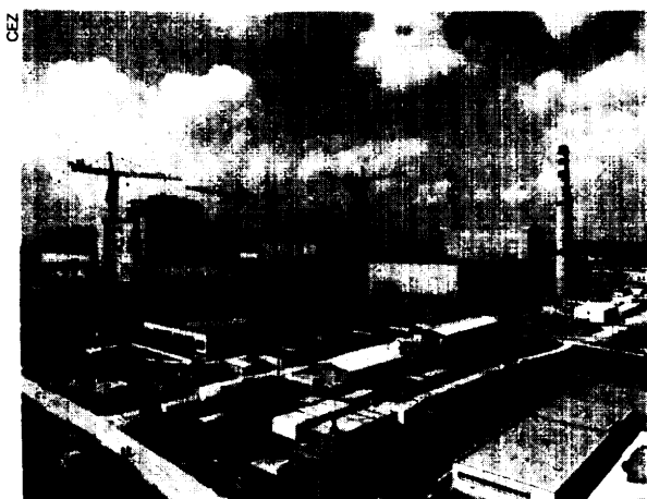
The Temelin Nuclear Powerplant, a VVER-1000 under construction in the Czech Republic with major assistance by Westinghouse Electric Corp.
